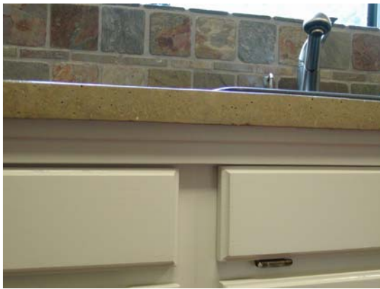
A piece of wood trim, painted to match the cabinets, is used to conceal the plywood substrate. Other treatment options are paint or metal trim.
