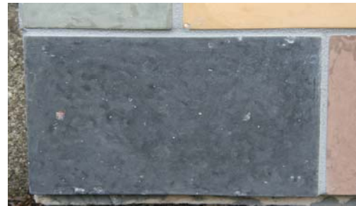
Worm holes in the surface of this tile were filled in by the grout when the joints were done.
