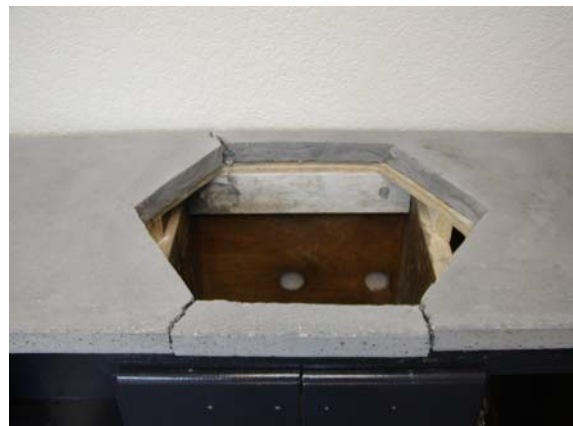
This slab broke from lack of experience.
