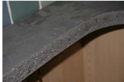
Undermount sink openings can have small air holes, formed during casting. These can be filled in and the edges should be sealed.
